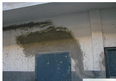
La Resurrection School buildings being repaired.
